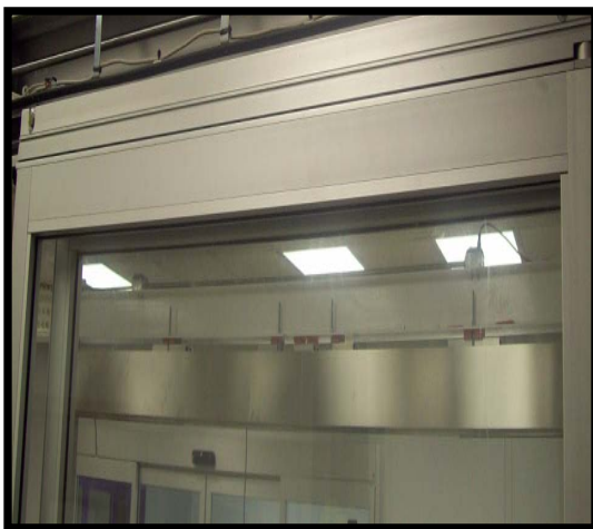
Slide open, release flush bolt & swing out
