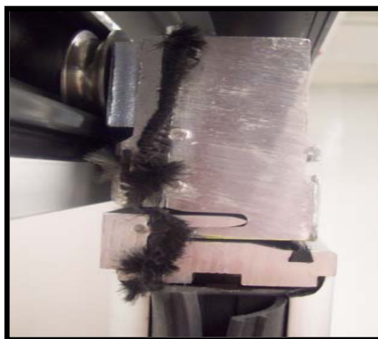
Slide open, release flush bolt & swing out
