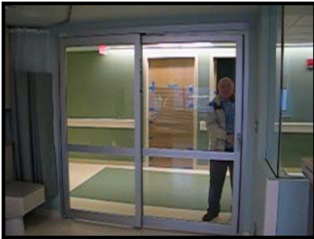
Slide open, release flush bolt & swing out
